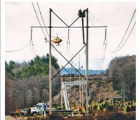
IBEW Local 42 and McPhee Electrical Contractors are building a new substation in Chicopee, MA.
